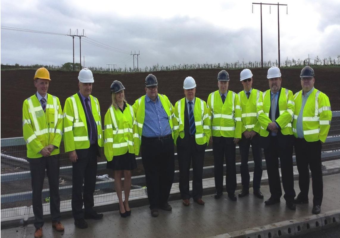
Members of the Committee for Regional Development at the site of the newly constructed A8 Belfast to Larne Dual Carriageway.
