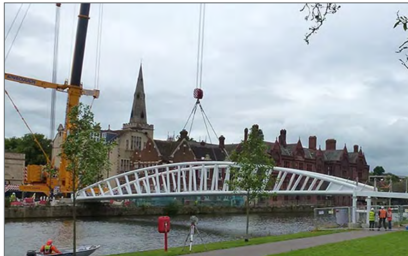
Figure 1-14: Example of Crane Erection of 4m Wide Prefabricated Pedestrian/Cycle Bridge Deck
