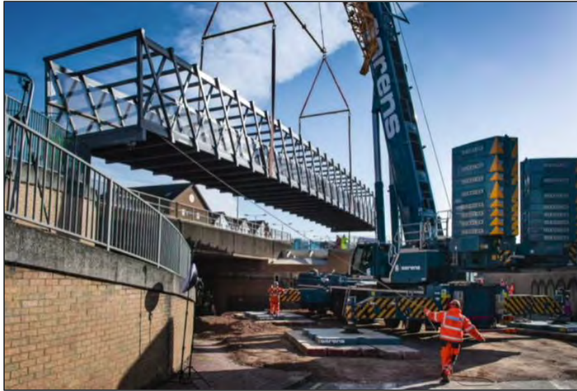
Figure 1-15: Example of Crane Erection of 4m Wide Prefabricated Pedestrian/Cycle Bridge Deck
