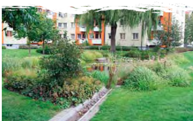
Augustenborg, Malmo, Sweden – an open channel leading from an unfenced amenity pond in a housing retrofit SuDS scheme. Photo: Bob Bray
