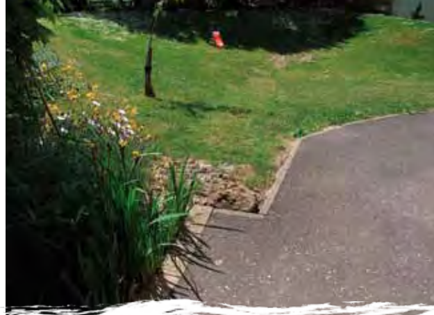
Springhill Housing, Stroud – a multi-functional detention basin and play space at the end of the management train that only fills after heavy rain. Photo: John Day (rspb)
