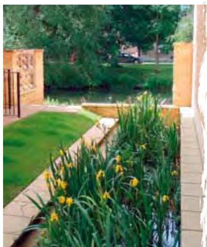
Riverside Court, Stamford – a canal as the final link in the management train, beginning with permeable paving, providing storage, amenity and biodiversity next to the River Welland. Photo: Bob Bray
