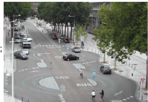
Figure 3: Example of cut through roundabout
