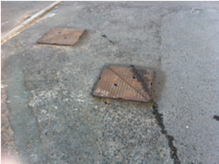
Drumbeg Mews - raised manhole covers
