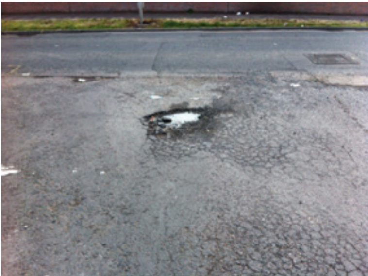
Drumbeg Mews - pothole
