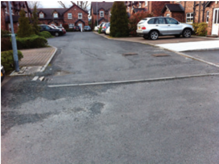
Drumbeg Mews - wide shot of uneven road surface
