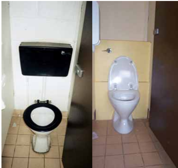
Case Study Figure: Old 9 litre toilets (on the left), replaced by new 4.5 litre toilets (on the right). Photos provided by Southern Water
