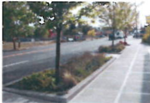
Tree Pit / Porous Paving retro fitted to roadway
