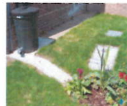
Water Butt to manage water at a local level
