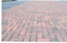
Permeable Paving (Marks & Spencer, Abbey Centre, NI)
