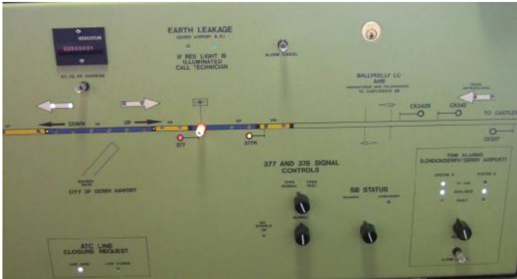
Figure 2.13 City of Derry Airport interface Panel at Londonderry Signalbox
