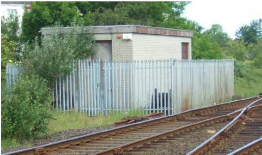
Figure 2.3 Coleraine Relay Room
