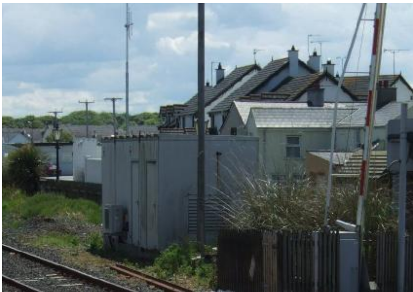
Figure 2.7 View of Castlerock REB from Signalbox
