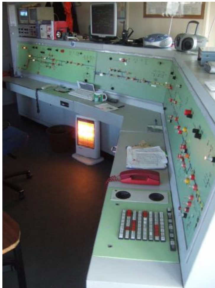
Figure 2.1 N-X panel at Coleraine Signalbox
