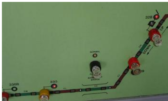
Figure 2.17 Release control Coleraine Signalbox
