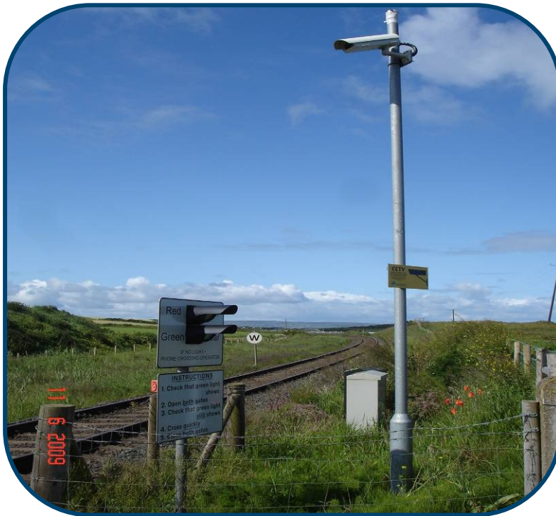
Figure 12: CCTV at Menarys UWC XP245 on Coleraine to Portrush line
