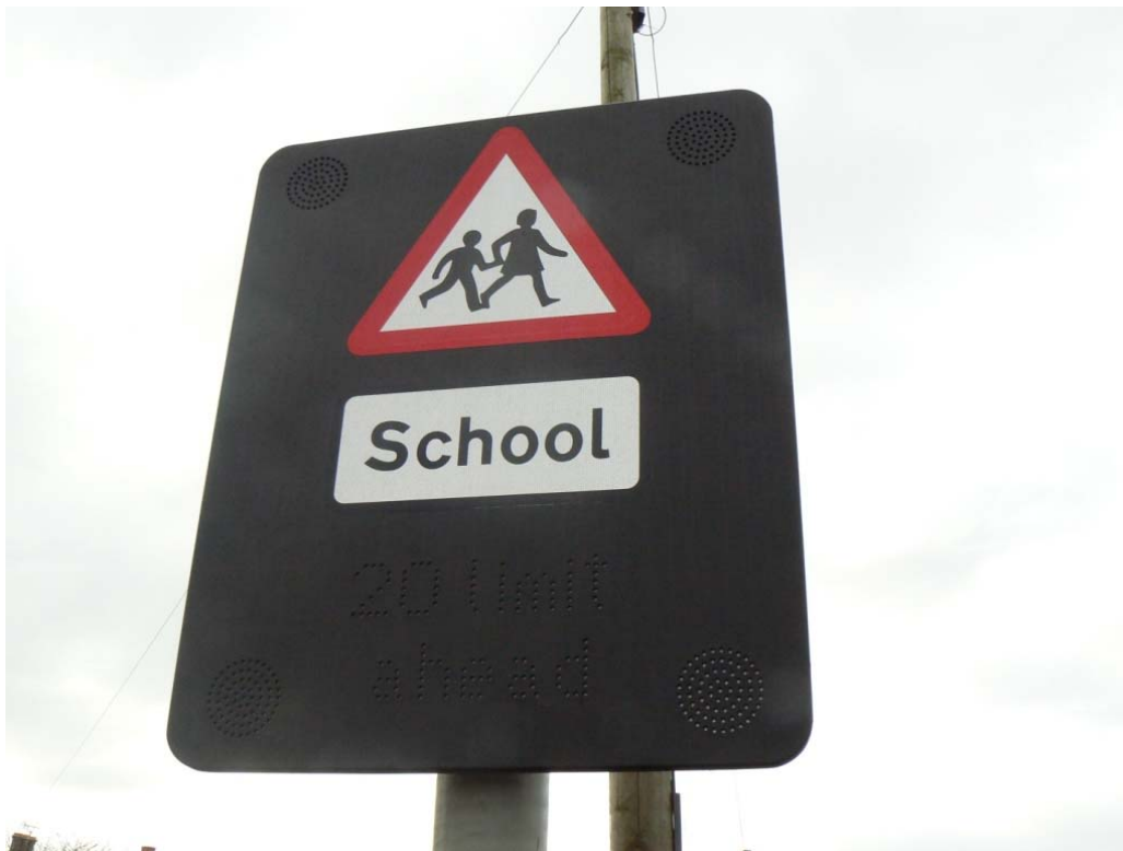
Rural solar powered Advance Slave Unit on local authority road (Aberdeenshire)
