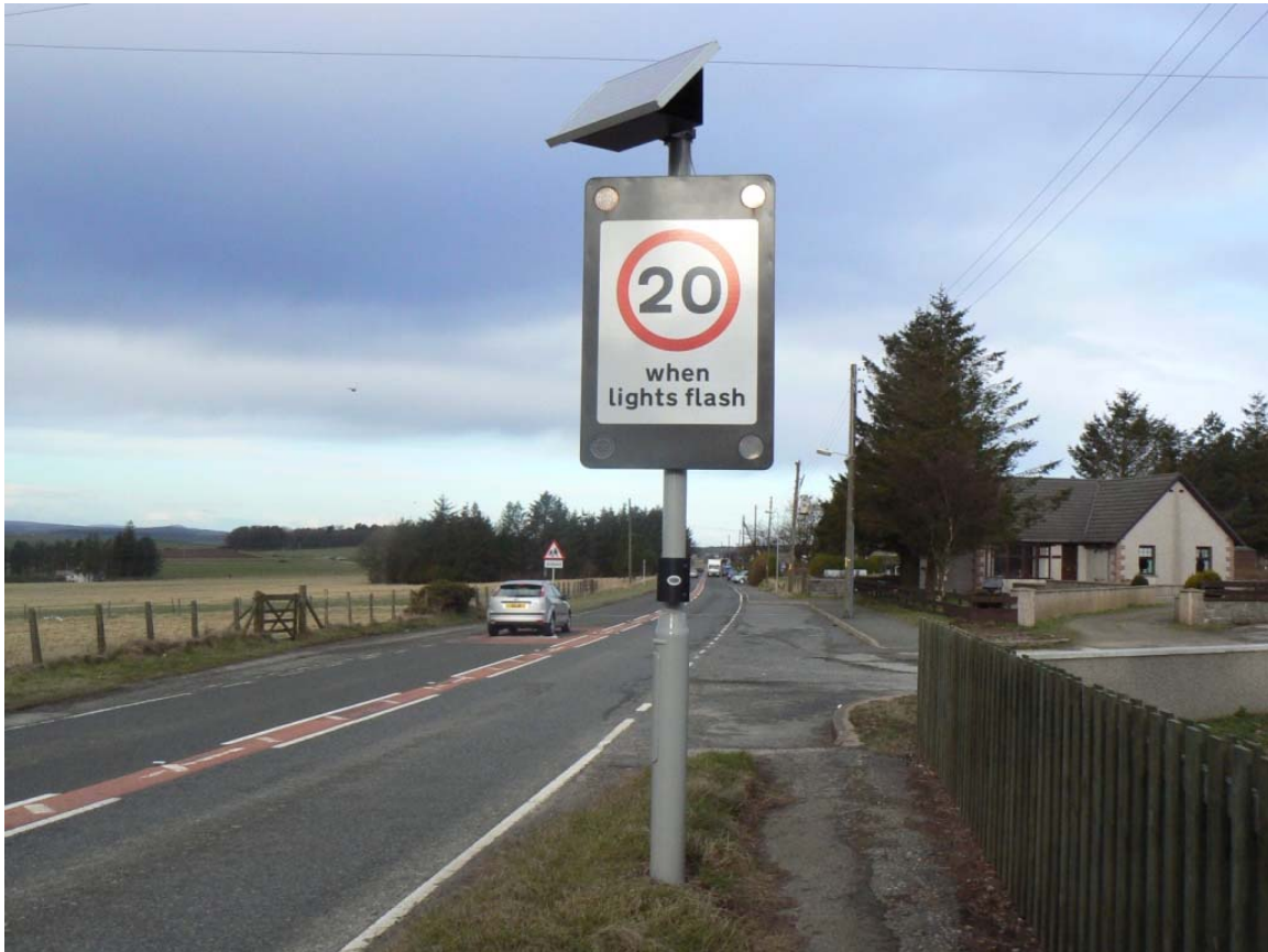
Rural solar powered speed limit sign on local authority road (Aberdeenshire)
