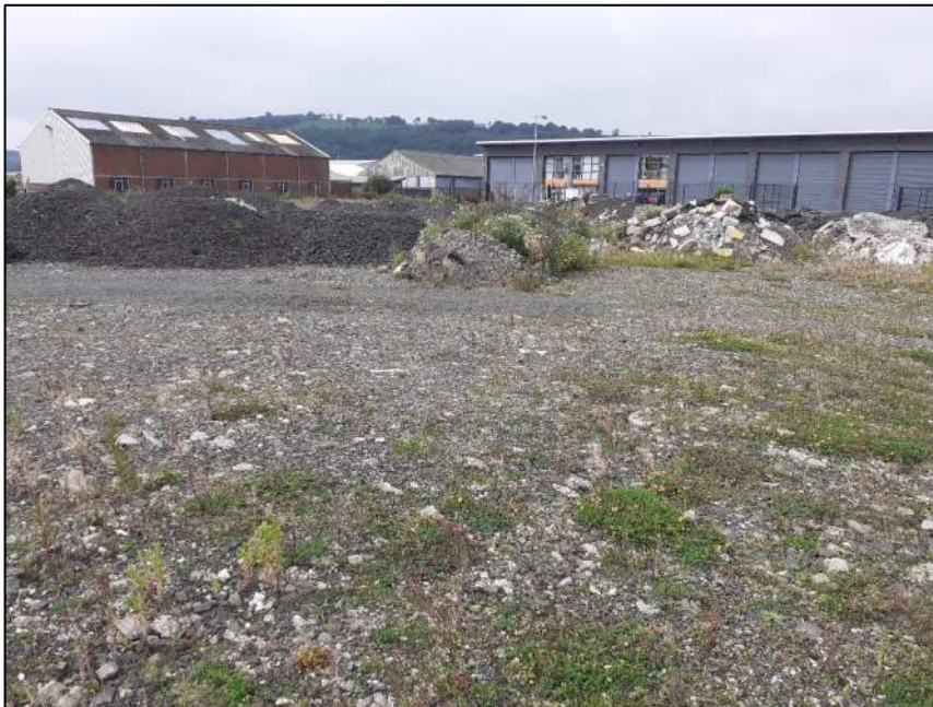
View of the stockpiles of gravel and demolition rubble at the western site boundary.
