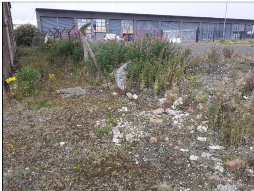
View at the rear of the former garage, to the west, showing the level change and the commercial units bordering the site to the west.
