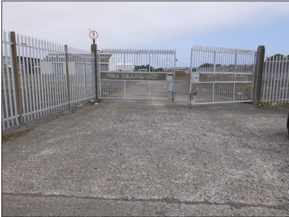
View of the entrance into the port owned section of site.
