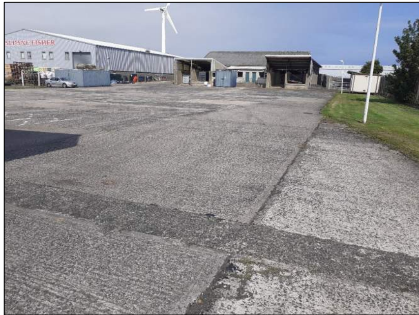
View to the north, behind the inspection centre building, of the lairage facility.
