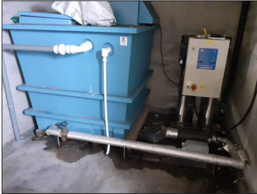
View of compressor and pump in the lairage for the power hosing.
