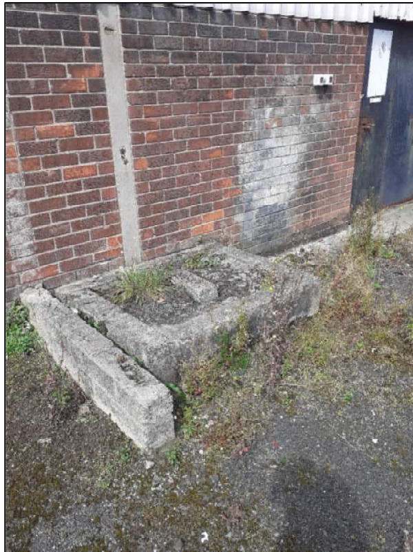
View of the remains of a brick base that may have housed a tank or boiler house.
