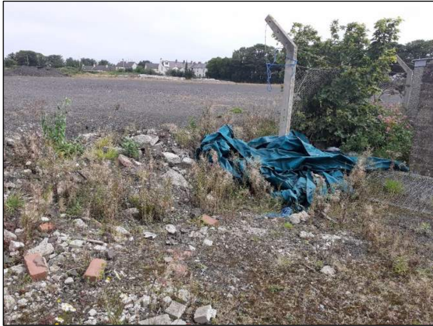
View of the rise in level from the southern section of the site to the mid site area and demolition wastes present.
