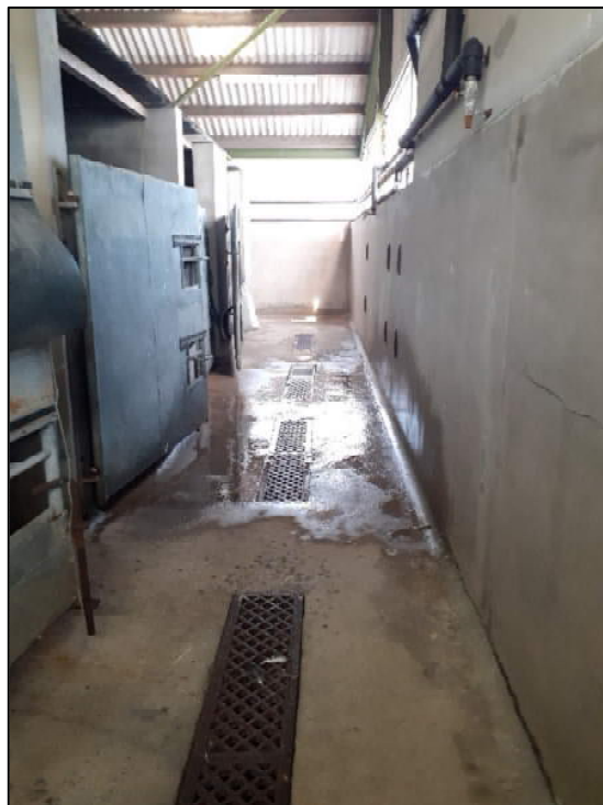
View inside the lairage showing drainage gates and hose on wall for washing down.
