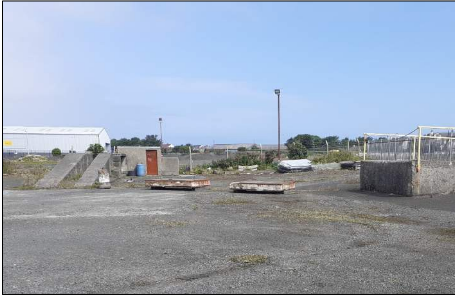
View of the vehicle inspection ramp with pump house to rear and viewing platform in the east.
