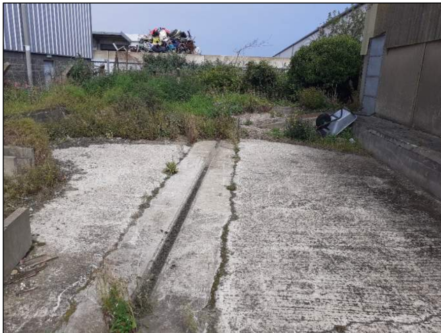
View to western side of lairage where used straw is dumped.
