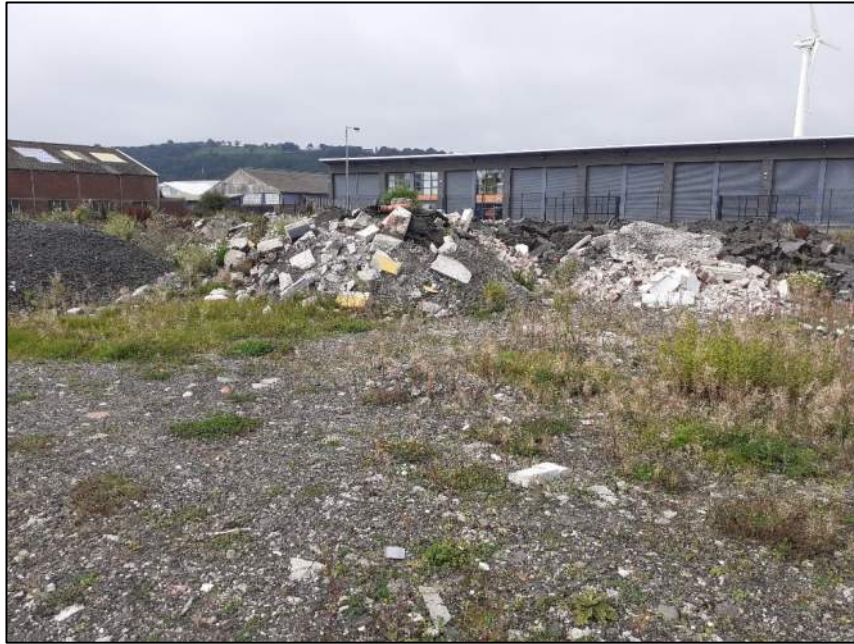
View of the demolition rubble stockpiles.
