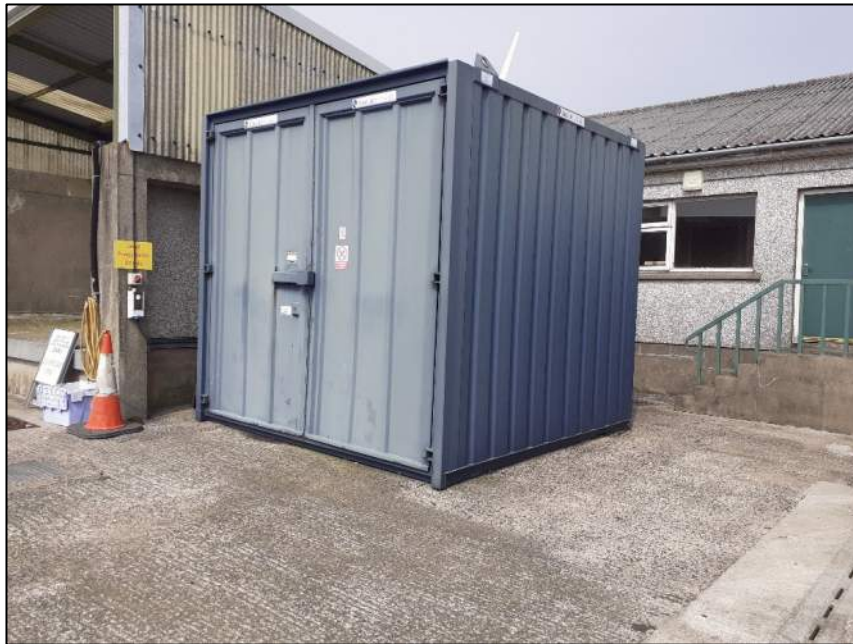
View of diesel tank and pump in container beside lairage.
