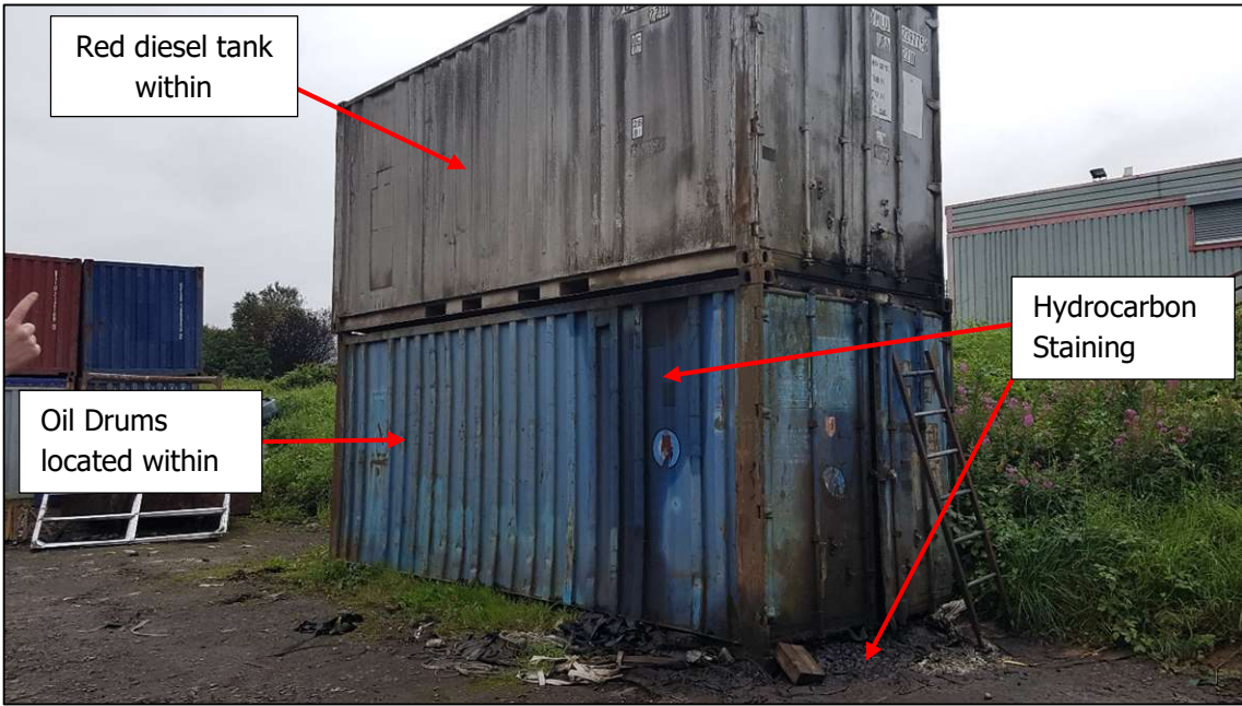
View of two containers located along the western boundary
