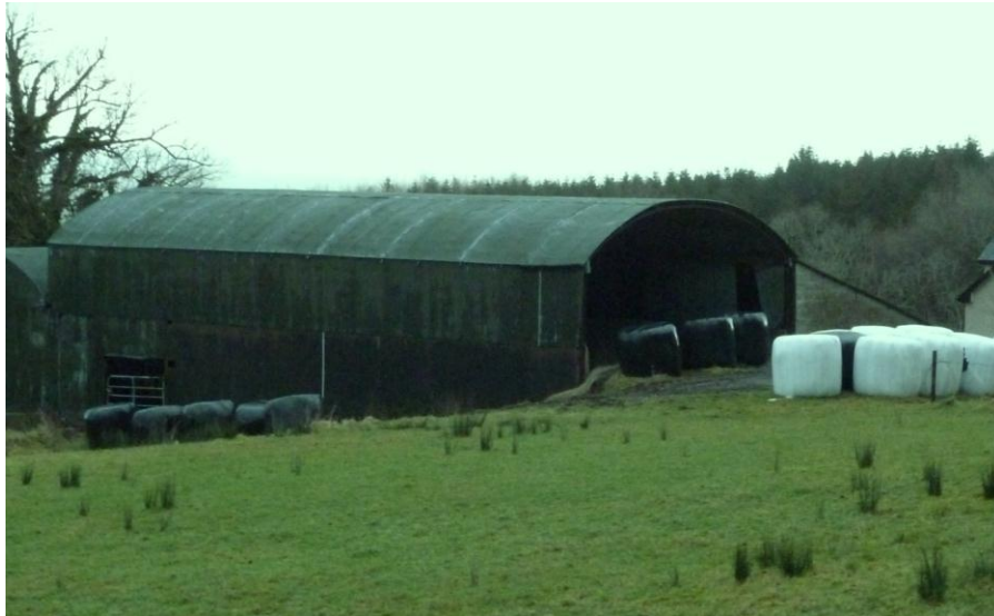
Irish barn compared to a compressor station in Alberta
