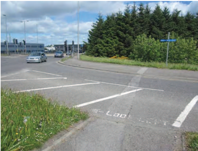
Looking north across Souter Head Road entrance from Souterhead roundabout
