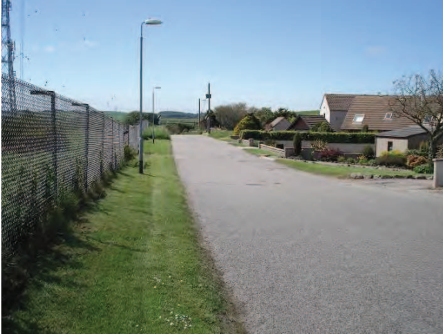
Redmoss Road looking south towards proposed site (left of image)
