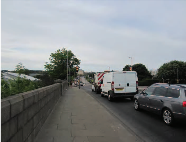
Wellington Road at bridge looking south
