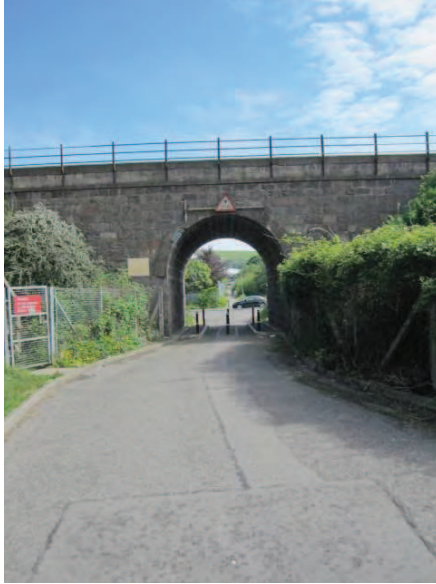
Rail underpass from Kirkhill Place, Torry, to Greenwell Road
