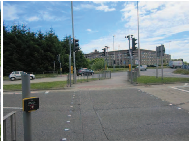
Toucan crossing across Wellington Road, north of Souterhead roundabout
