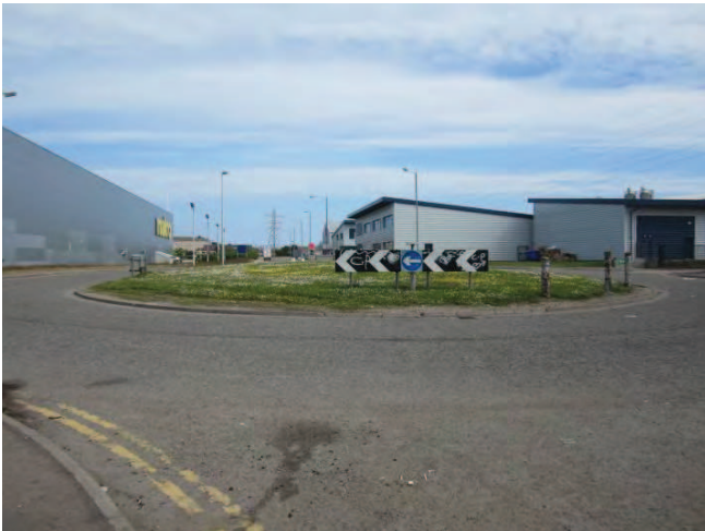
Roundabout at end of Wellington Circle, looking east
