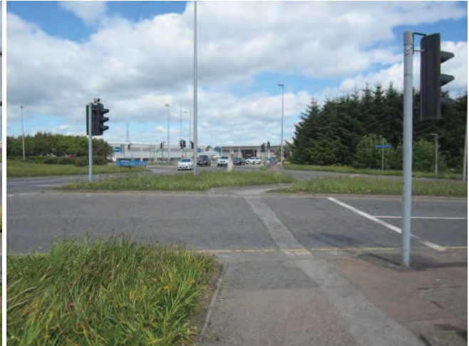
Looking north-west across Souter Head Road exit onto Souterhead roundabout
