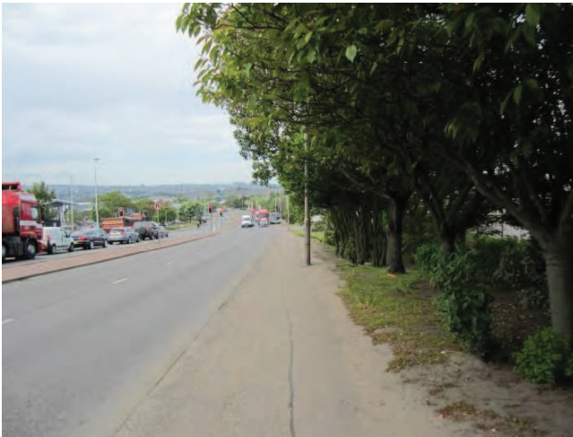
Wellington Road near Altens Farm Road looking north
