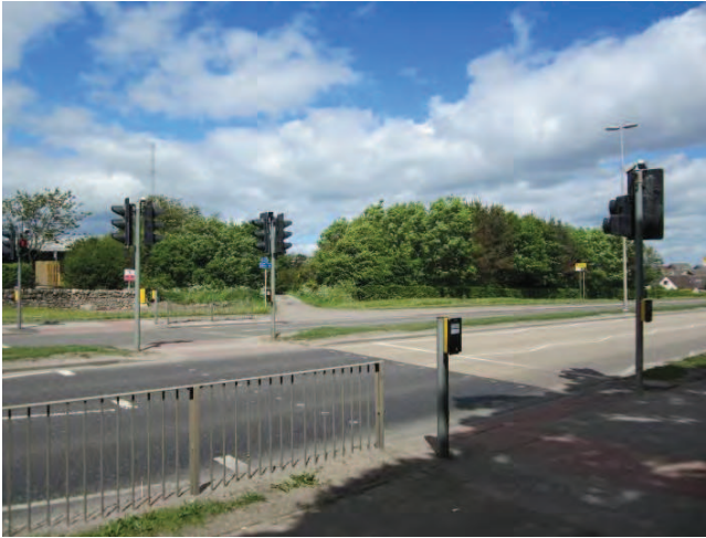
Signalised crossing point, looking north east over Wellington Road
