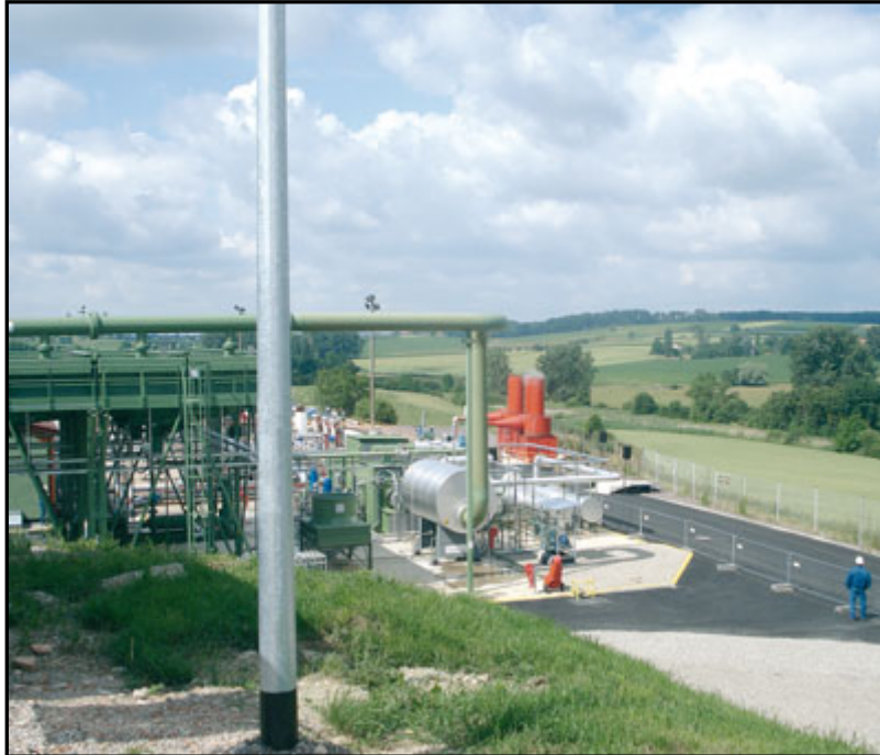
Figure 2: The Soultz geothermal power plant
