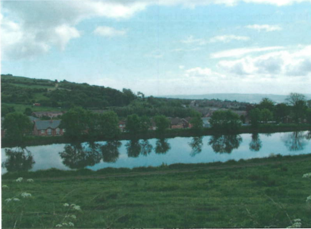
1. View of Wolfhill Middle Dam from the Wolfhill Upper Dam.
