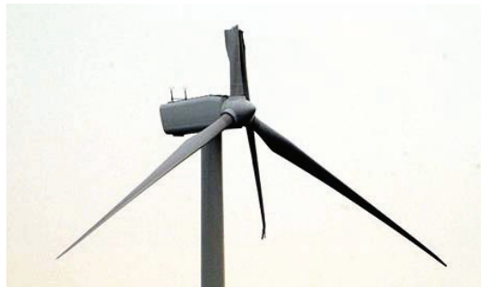
Figure 2 Example of a mid-span blade failure
