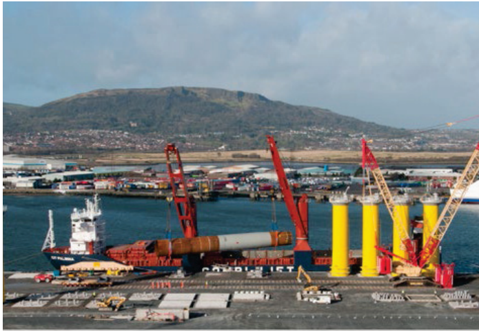
It took 15 months to build Belfast's new offshore wind terminal. Image supplied by DONG Energy.
