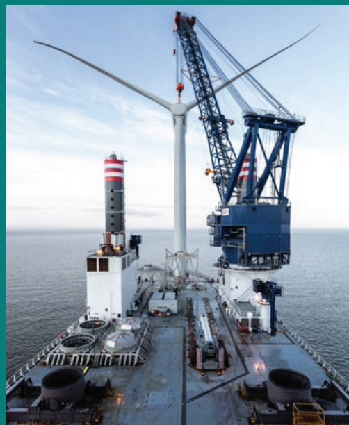
Attaching blades to rotor
