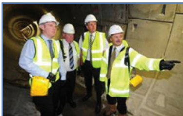
Committee Members on a visit to the Belfast sewers project.
