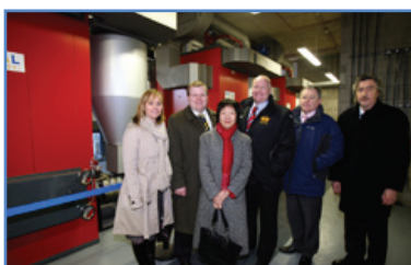
Members of the Committee receive a briefing on eco-friendly district heating systems during their visit to the eco village in Lisburn.
