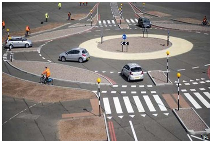
Figure 4: A typical Dutch roundabout built by the Transport Research Laboratory at its facility in Berkshire (see photo above) with a view to rolling out the design in key locations in London in 2015
