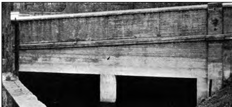
Fig.8 Photograph of widened downstream elevation of Saltwater Bridge, 1936 (Millin 1938).
