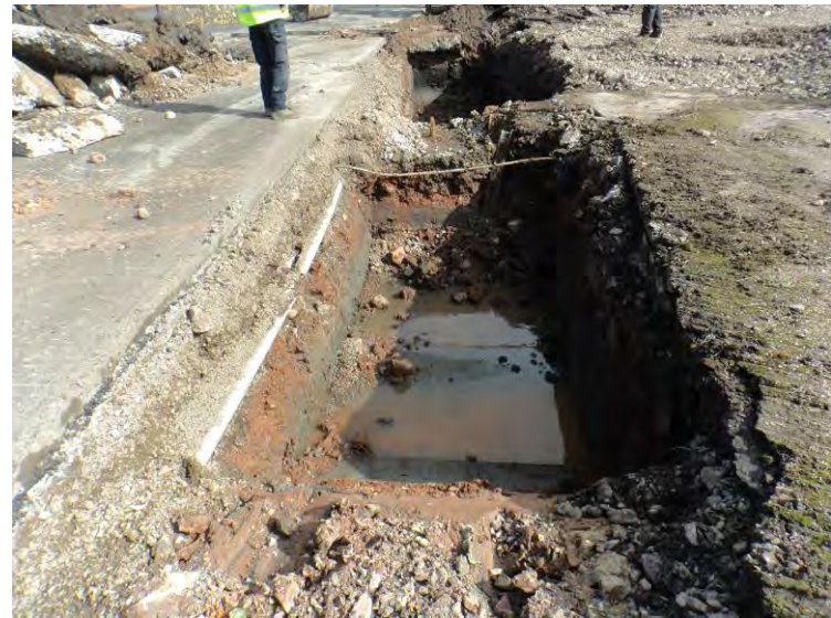
Plate 8 Trench 5, plastic ducting visible, facing northeast.
