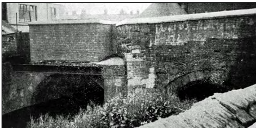
Fig.6: View of east face of Salt-water Bridge, c.1934 (Millin, 1938).
