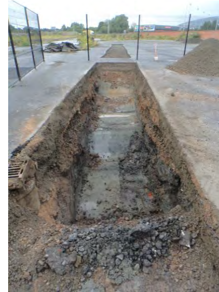
Plate 4 Trench 2, facing southwest.
