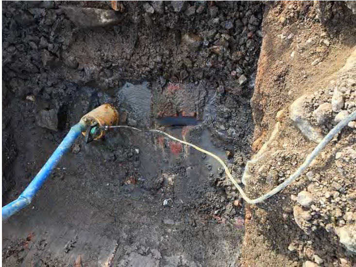
Plate 5 Trench 3, brick drain C14, facing southwest.
