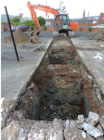
Plate 7 Trench 4, facing northwest.
